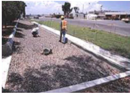
a) Infiltration Trench – Parking lot
