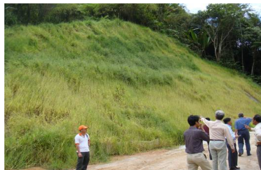
b) Completed Hydroseeding
