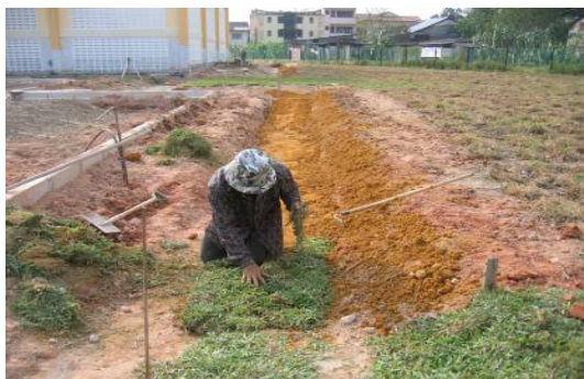
a) Turfing in Progress
