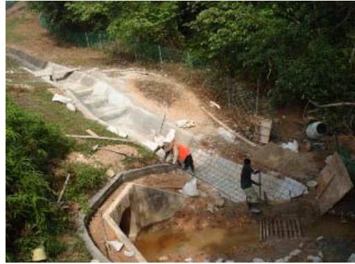
Figure AX2.10: Maintenance Work for Culvert
