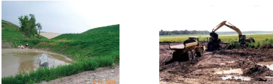
Figure AX2.6: Sediment Removal Work
