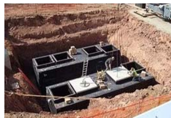
d) Oil and Grease Interceptor - Type 3
