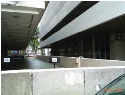
Floodwalls with entry and exit gates
